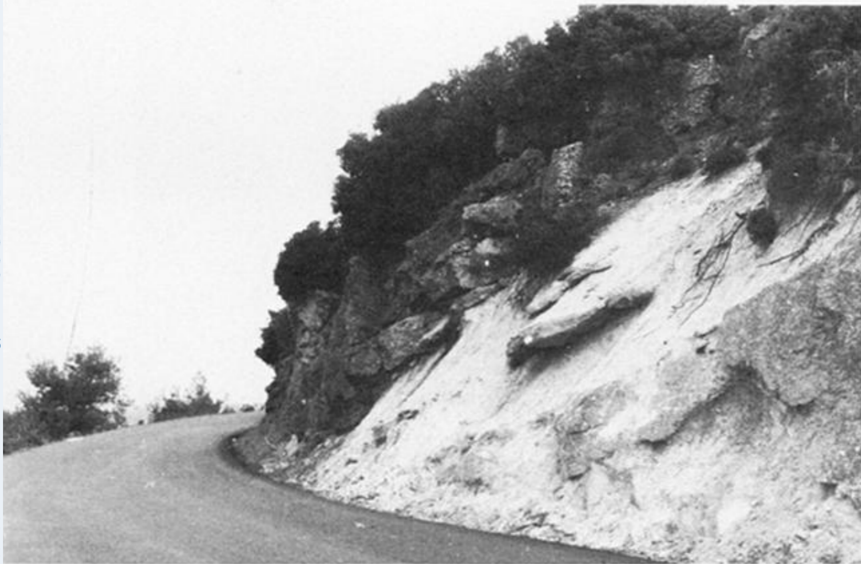
FIGURE 15. Folding of the caprock over a buried fault on the Kiaton road (see A in figure 14). The caprock is composed of sands and gravels of continental origin. In some places it is clearly fluvial. In general the composition is coarser and the caprock thicker (up to 3 m) near the hills, and it becomes finer and thinner near the coast where it is also mixed with beach deposits. The caprock results from the transgression of debris from the adjacent mountains over the marls as the sea or lake in which they were deposited retreated. In some places (including this location) marls are interbedded with the caprock near the surface indicating that the retreat was not monotonic. Caprock covers the marls and is conformable with the land surface except where it has been removed by badland erosion or where limestone outcrops rise above the old lake surface (see figure 11).
